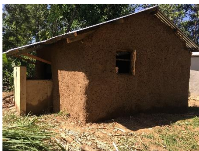
Fig. 6. Prototype kitchen with an exterior placement of the cooking stove. The new design eliminates smoke build-up inside the kitchen almost completely.
